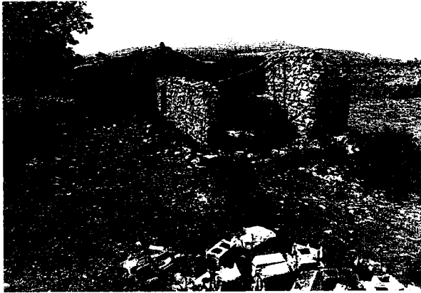
Plate 3. VG1 viewed from south-east; note modern breeze-blocks in foreground
